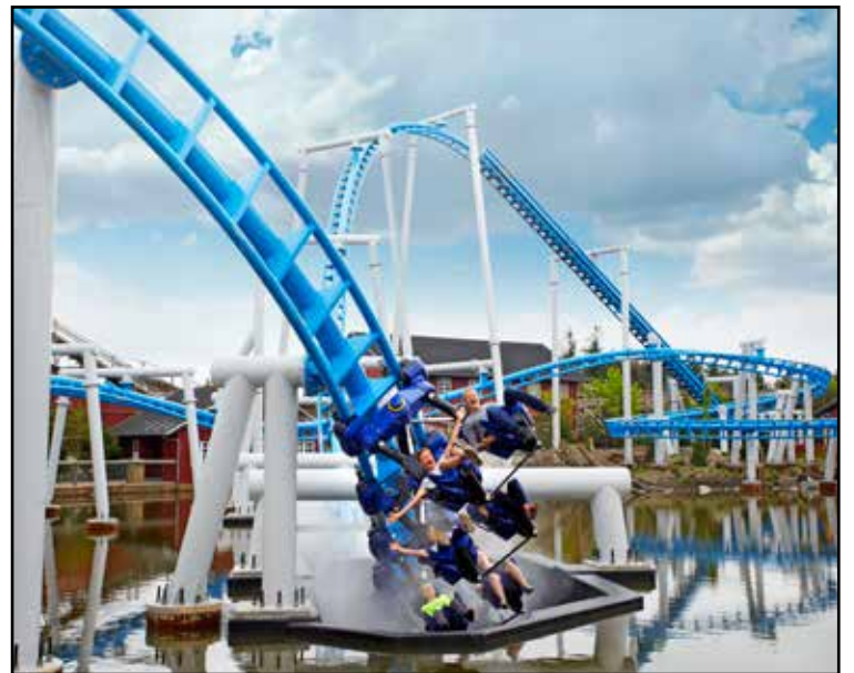
Faarup Sommerland's 2013 season is highlighted by the opening of the Hurricane, a custom-designed Family Suspended Coaster supplied by Vekoma. The 1,486-foot-long coaster features a number of unique attributes including an underwater tunnel, an overbanked horseshoe, two horizontal loops and numerous changes in direction.
