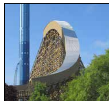
Noise-mitigation efforts on Gold Striker include a 174-foot first-drop tunnel incorporated into its original design and a late-added 70-foot midcourse tunnel that necessitated the coaster’s sudden two-day closure in early July. COURTESY CALIFORNIA’S GREAT AMERICA
