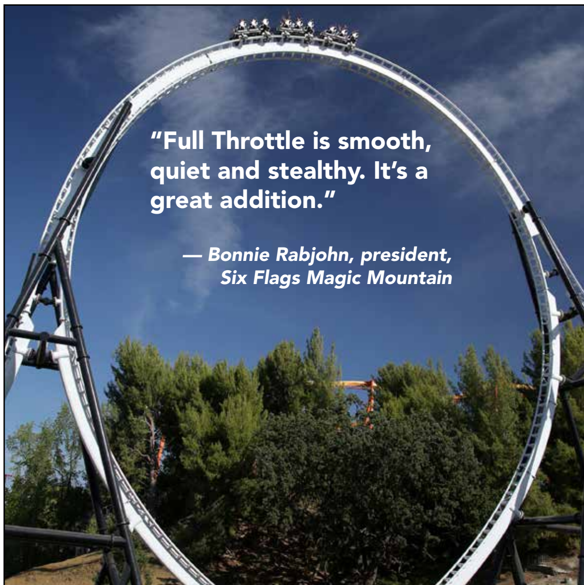
Several views (above and below) of Full Throttle cresting the outside of its record-setting, 160-foot-high loop just before the train returns to the station. This one-of-a-kind, loop-capping "top hat" element is made possible by consecutive reverse and forward midcourse LSM launches after the initial 70-mph LSM launch.
