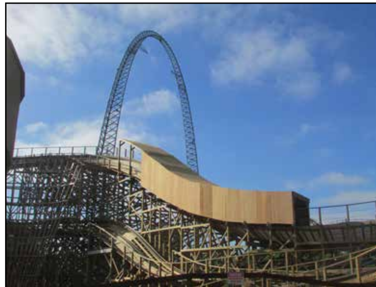
Noise-mitigation efforts on Gold Striker include a 174-foot first-drop tunnel incorporated into its original design and a late-added 70-foot midcourse tunnel that necessitated the coaster’s sudden two-day closure in early July. COURTESY CALIFORNIA’S GREAT AMERICA
