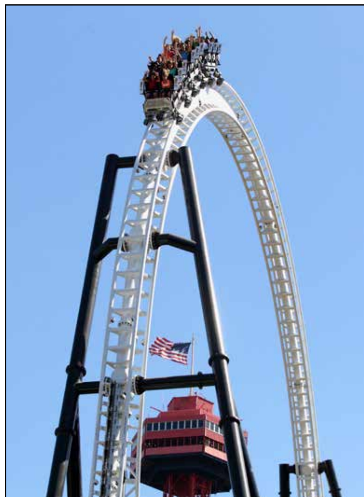
Several views (above and below) of Full Throttle cresting the outside of its record-setting, 160-foot-high loop just before the train returns to the station. This one-of-a-kind, loop-capping "top hat" element is made possible by consecutive reverse and forward midcourse LSM launches after the initial 70-mph LSM launch.
