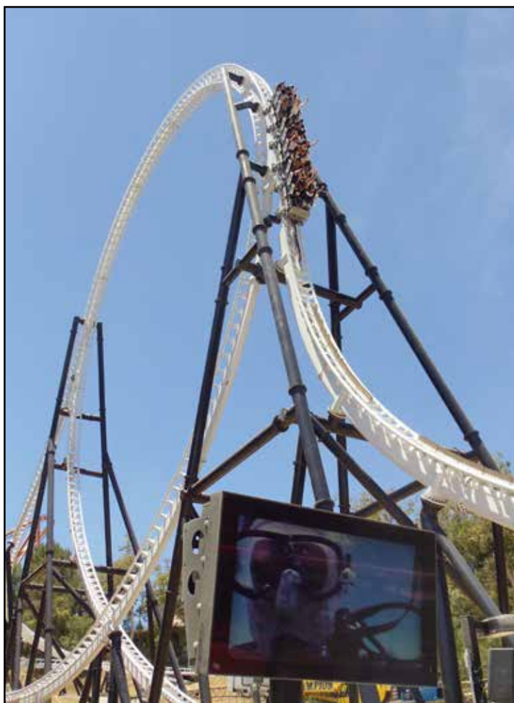
Several views (above and below) of Full Throttle cresting the outside of its record-setting, 160-foot-high loop just before the train returns to the station. This one-of-a-kind, loop-capping "top hat" element is made possible by consecutive reverse and forward midcourse LSM launches after the initial 70-mph LSM launch.
