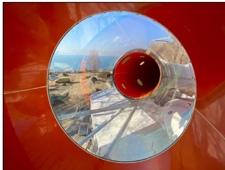
A Wiegand tube slide includes a clear acrylic section (above) to give riders a surprise view of the surrounding lake. Most of the slide structure is located outside the main building. The clear acrylic section and light stripes are seen at right.
