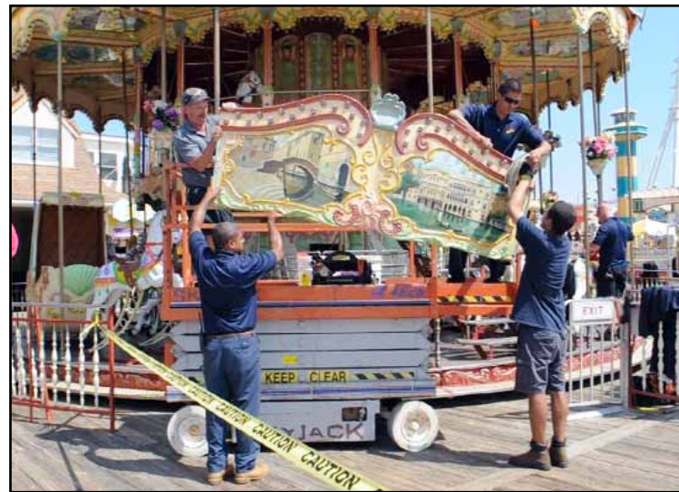
Morey's Piers, in Wildwood, N.J., did not suffer major damage from the east coast storms, but did lose some business due to the closed days. Here workers begin the process of putting the park back together for reopening. COURTESY MOREY'S PIERS
