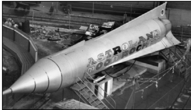
The Astroland Moon Rocket sat surrounded by construction debris as the park took shape.
