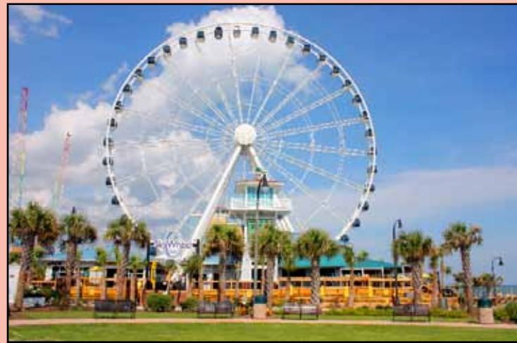
The SkyWheel at Myrtle Beach Landing — a new Chance Morgan R60 Giant Wheel — debuted this spring. The 187-foot-tall ride features 42 glass-enclosed, temperature-controlled gondolas that hold up to six passengers each. AT/SCOTT RUTHERFORD
