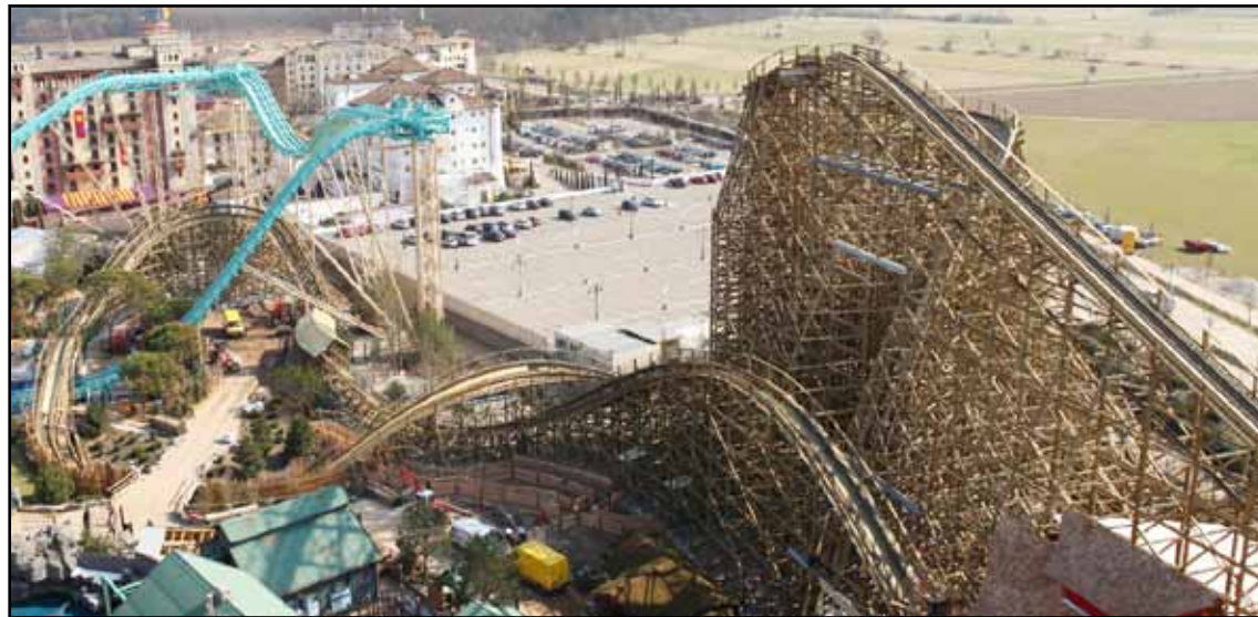
Wodan's massive support structure was constructed with timber acquired from sustainable German forests while the laminates for the 3,445-foot-long wooden track were imported from the U.S. COURTESY EUROPA-PARK
