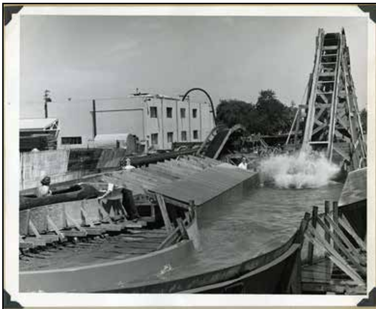
Testing of the world’s first log flume as seen at Arrow Development’s Mountain View, California facility. COURTESY NATIONAL ROLLER COASTER MUSEUM / RON TOOMER COLLECTION
