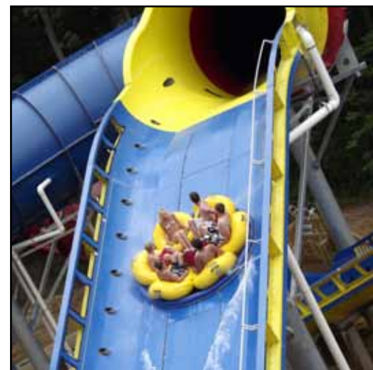
ProSlide used Holiday World's natural terrain in the design of Mammoth. The HydroMagnetic water coaster features 100 LIM's to power the rafts through the course providing a capacity of 1,000 pph. COURTESY PROSLIDE
