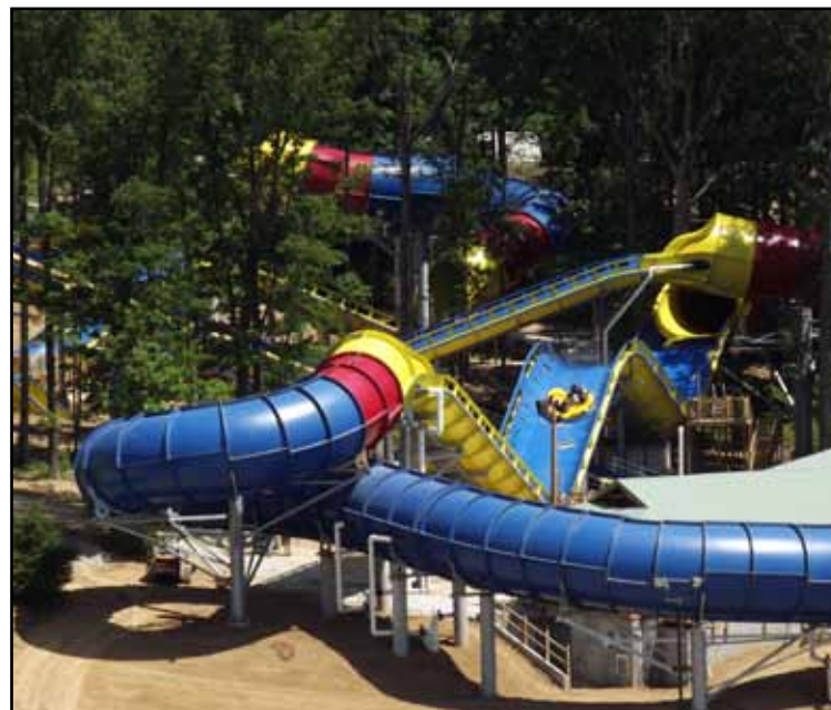
ProSlide used Holiday World's natural terrain in the design of Mammoth. The HydroMagnetic water coaster features 100 LIM's to power the rafts through the course providing a capacity of 1,000 pph. COURTESY PROSLIDE
