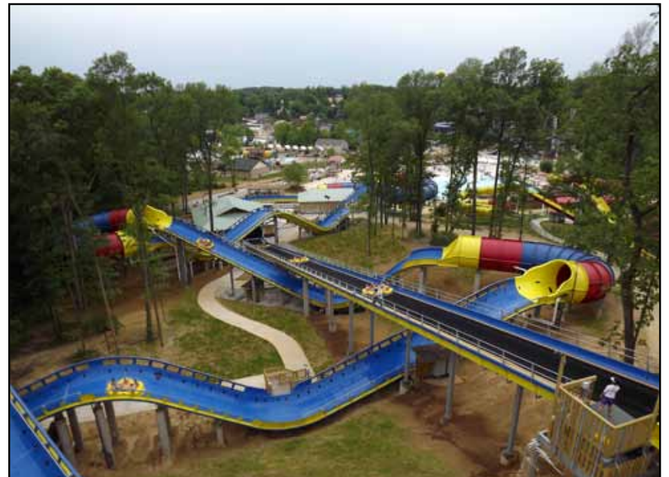
Holiday World & Splashin' Safari's new Mammoth HydroMagnetic water coaster from ProSlide is a record setter. The $9 million ride is the world's longest such ride at 1,763 feet, and uses 100 LIM's to blast the six-passenger rafts through the course. COURTESY PROSLIDE
