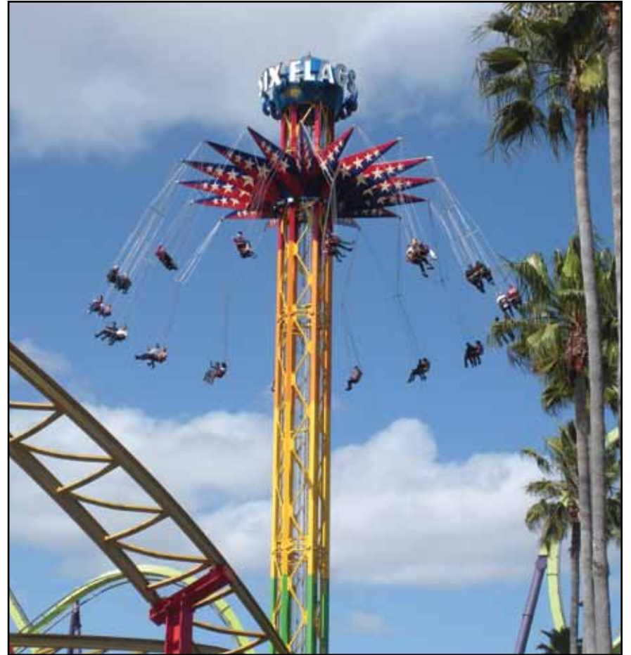
SkyScreamer, a 150-foot-tall, Funtime StarFlyer swing ride made its debut this spring at California's Six Flags Discovery Kingdom. The new ride, located on a new plaza inside the park's Medusa floorless coaster, seats 32 riders and helps to redefine the park's skyline. COURTESY RIDE ENTERTAINMENT GROUP
