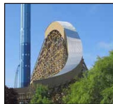
Noise-mitigation efforts on Gold Striker include a 174-foot first-drop tunnel (right) incorporated into its original design and a late-added 70-foot midcourse tunnel (above and below) that necessitated the coaster’s sudden two-day closure in early July. COURTESY CALIFORNIA’S GREAT AMERICA
