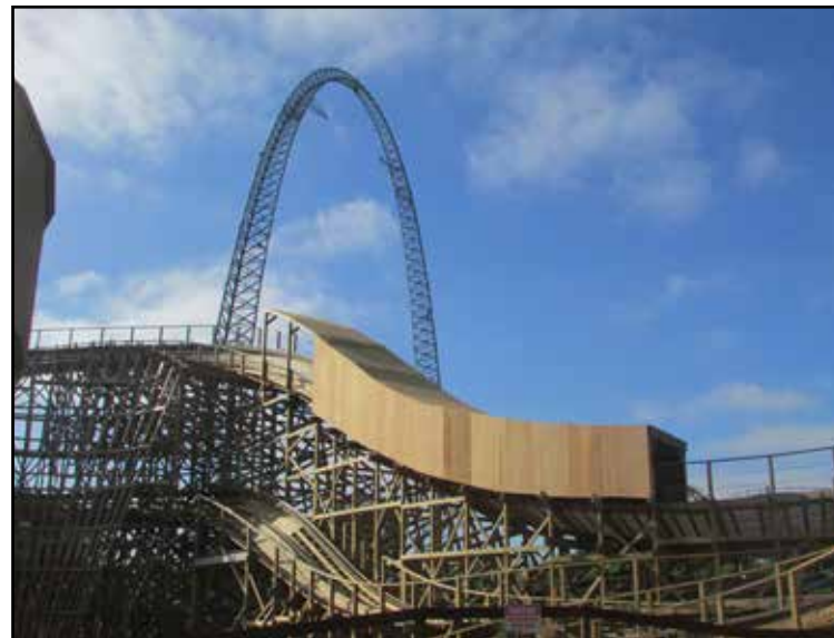
Noise-mitigation efforts on Gold Striker include a 174-foot first-drop tunnel (right) incorporated into its original design and a late-added 70-foot midcourse tunnel (above and below) that necessitated the coaster’s sudden two-day closure in early July. COURTESY CALIFORNIA’S GREAT AMERICA
