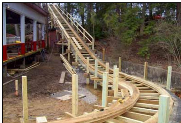
Idlewild Park's 1938-built Rollo Coaster is one of the latest wooden coasters to undergo major off-season rehab work. Following the original PTC blueprints, Idlewild's maintenance team completely rebuilt 250 feet of Rollo Coaster's course, which included foundations, track and structure from the coaster station, around the first curve and to the top of the lift hill. COURTESY IDLEWILD PARK
