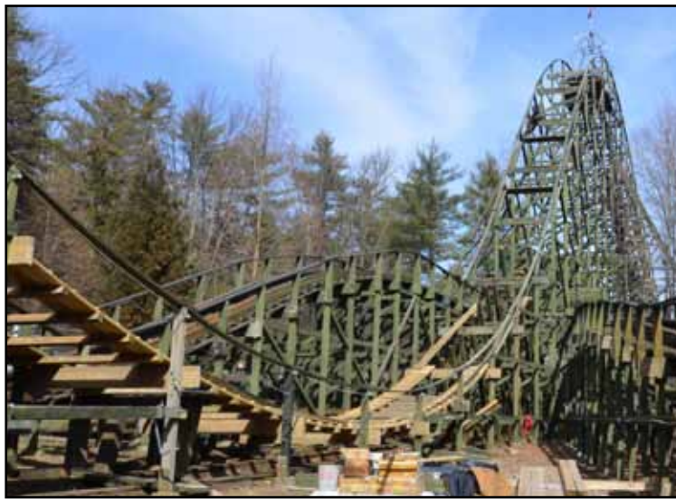
Knoebels popular Phoenix is getting 400 feet of new track coming off the lift hill and continuing through to the first turn. Structural Technologies is completing the work for the park. COURTESY KNOEBELS
