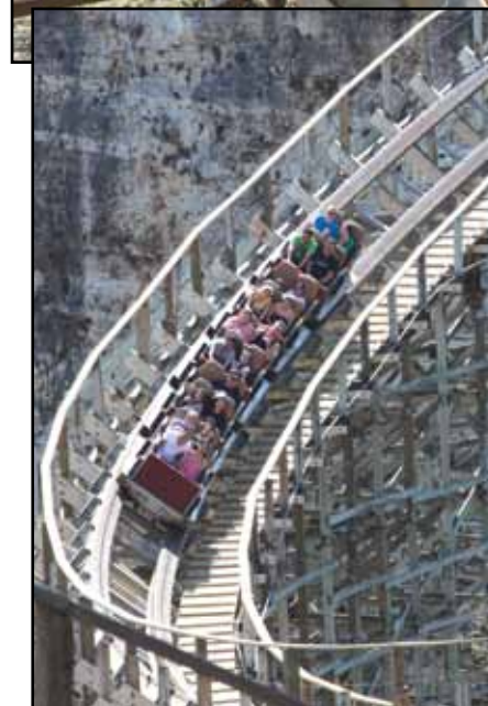
The Rattler wooden roller coaster at Six Flags Fiesta Texas is sporting 345 feet of new Topper Track this season, supplied by Rocky Mountain Construction. The Topper Track features six layers of glued wood with a steel box rail mounted on top of the wood base. The revamped section of track was on the ride's big curving drop into the quarry's bottom. AT / GARY SLADE
