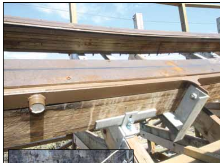
The Rattler wooden roller coaster at Six Flags Fiesta Texas is sporting 345 feet of new Topper Track this season, supplied by Rocky Mountain Construction. The Topper Track features six layers of glued wood with a steel box rail mounted on top of the wood base. The revamped section of track was on the ride's big curving drop into the quarry's bottom. AT / GARY SLADE
