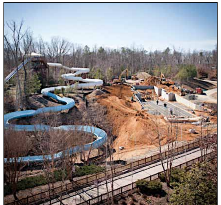
Construction began last fall on Water Country USA's new attraction, Vanish Point. Here is a view of the new feature under construction. COURTESY WATER COUNTRY USA
